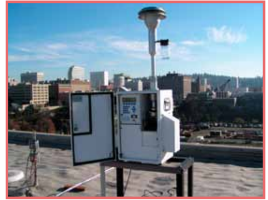
Air quality sampling stations are located on rooftops, as pictured here at the Spokane Regional Public Health Building
