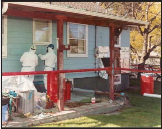
Prying to expose nail heads
