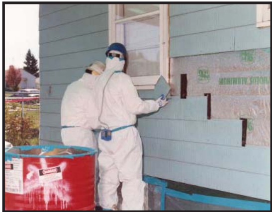
Removing siding
