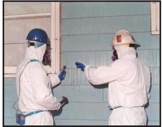
Pulling out nails
