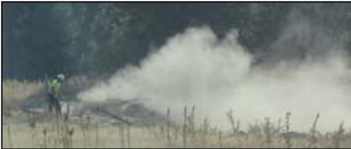
*Improper dust control using compressed air to clean cracks prior to sealing.*
