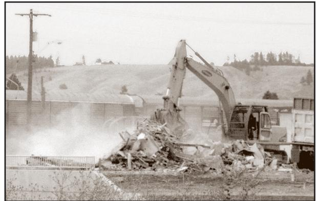
*Uncontrolled dust emissions come from a variety of commercial activities. Inhaling fine dust particles can be a health hazard as well as a public nuisance. Uncontrolled dust emissions can result in enforcement action and fines.*
