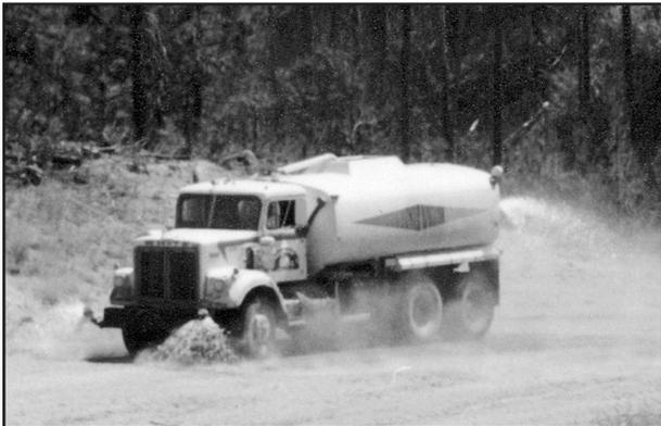
*Using water or a chemical dust suppressant is one way to minimize dust emissions.*
